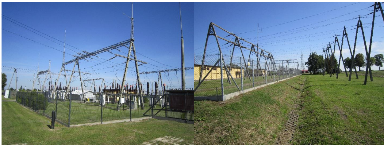
Fot. 4 i 5. GPZ Hrubieszów 110/30/15 kV
